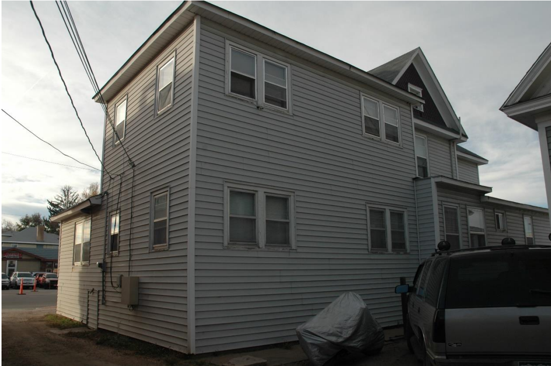
CD 1, Image 193, View to NW of east and south sides showing the 1920s addition
