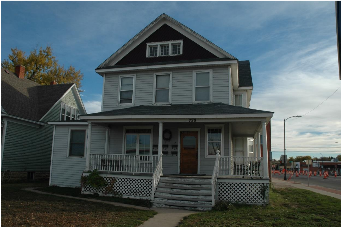
CD 1, Image 194, View to south of façade (north)
