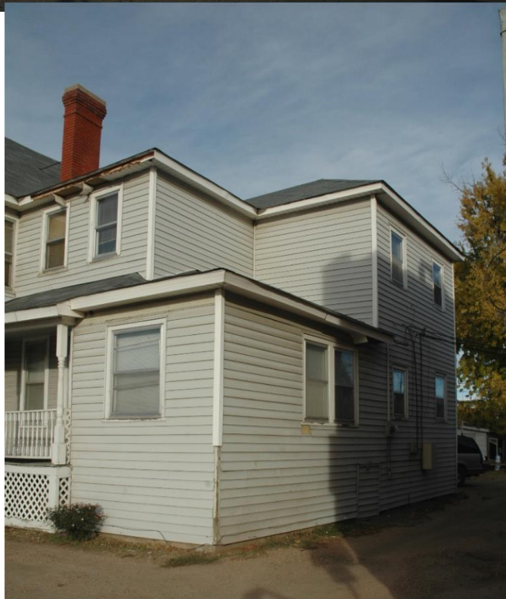
CD 1, Image 192, View to NE of south side and SW corner
