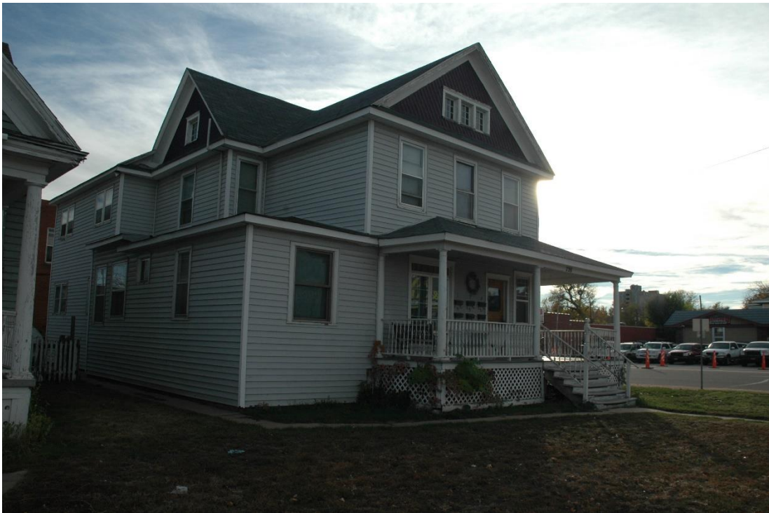
CD 1, Image 195, View to SW of façade (north) and east side
