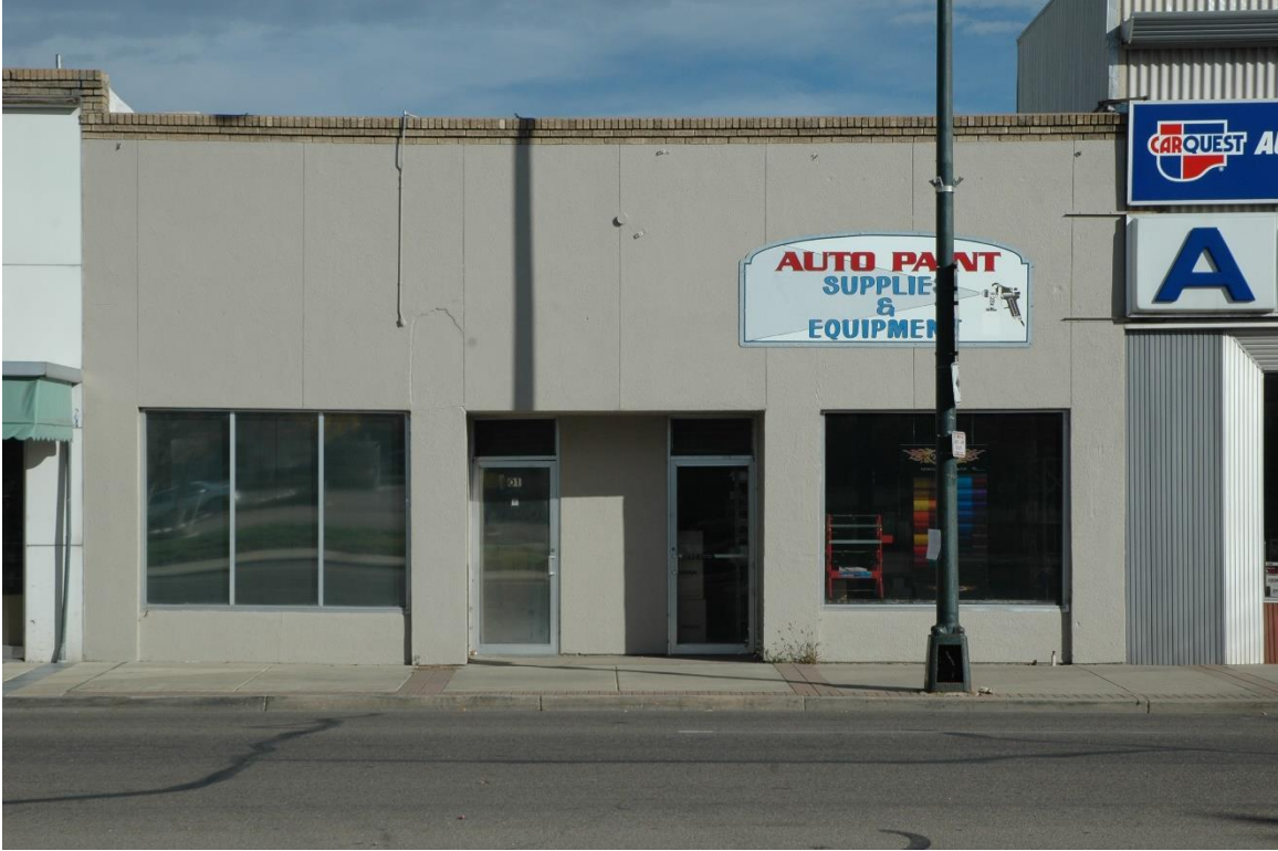
CD 1, Image 137 View to east of façade (west)
