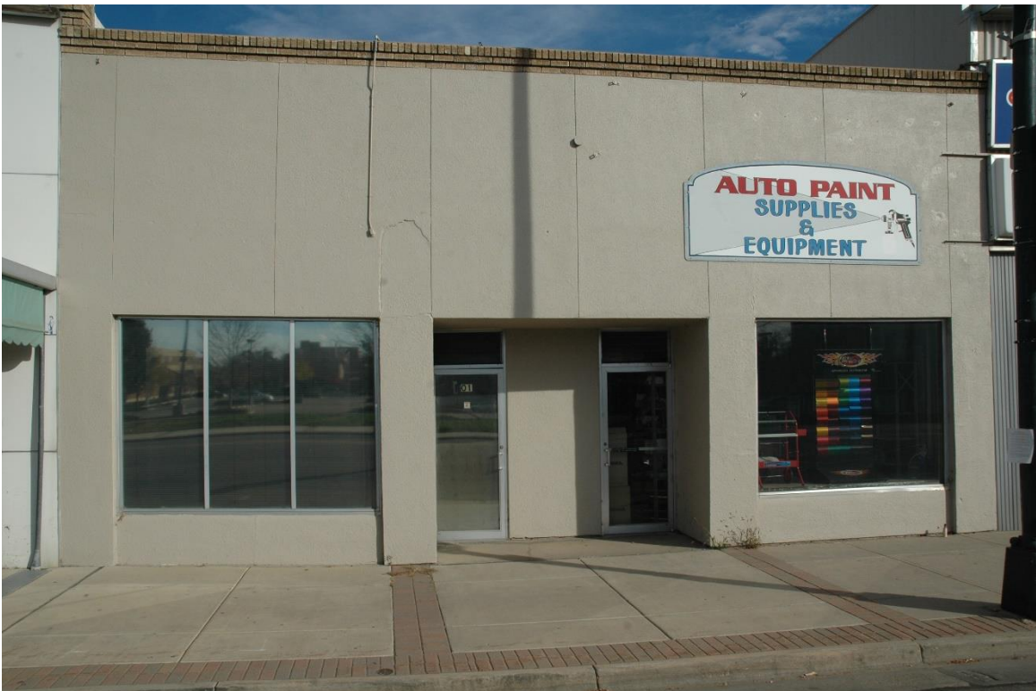
CD 1, Image 146, View to east of façade (west)
