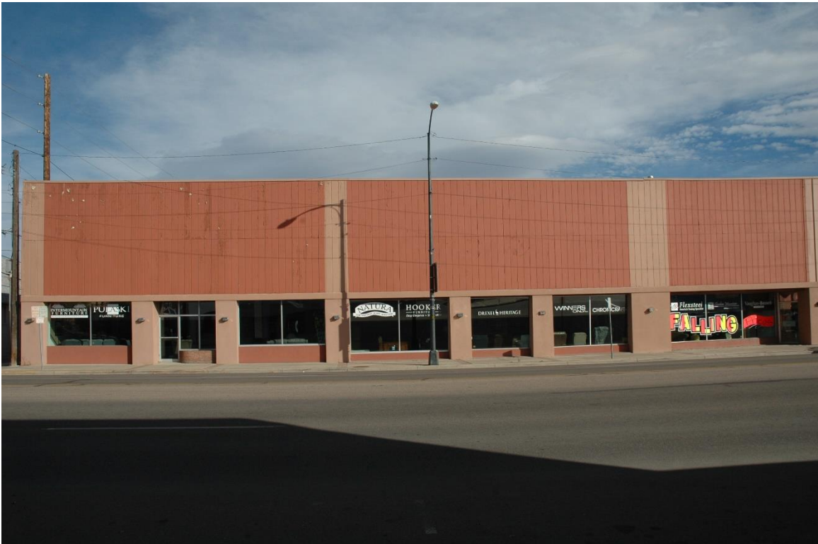
CD 1, Image 141, View to east of façade (west)
