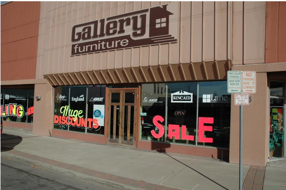
CD 1, Image 154, View to ENE of storefront and entry door on facade
