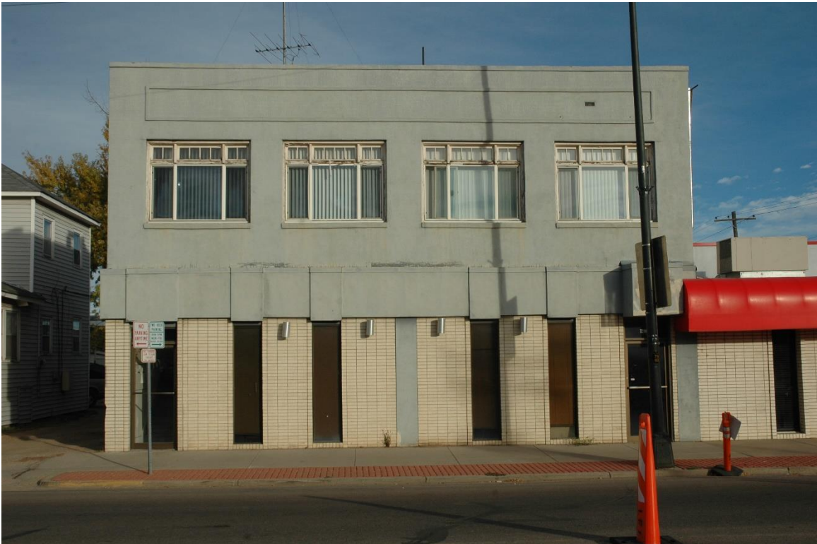
CD 1, Image 197, View to east of façade (west)
