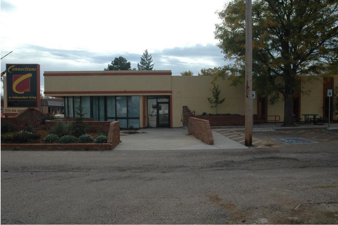
CD 1, Image 75, View to south of north side
