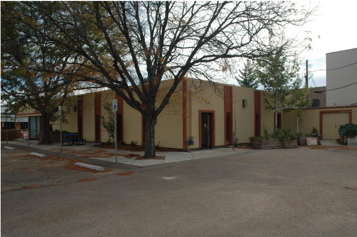
CD 1, Image 76, View to SE of north side and rear (west)
