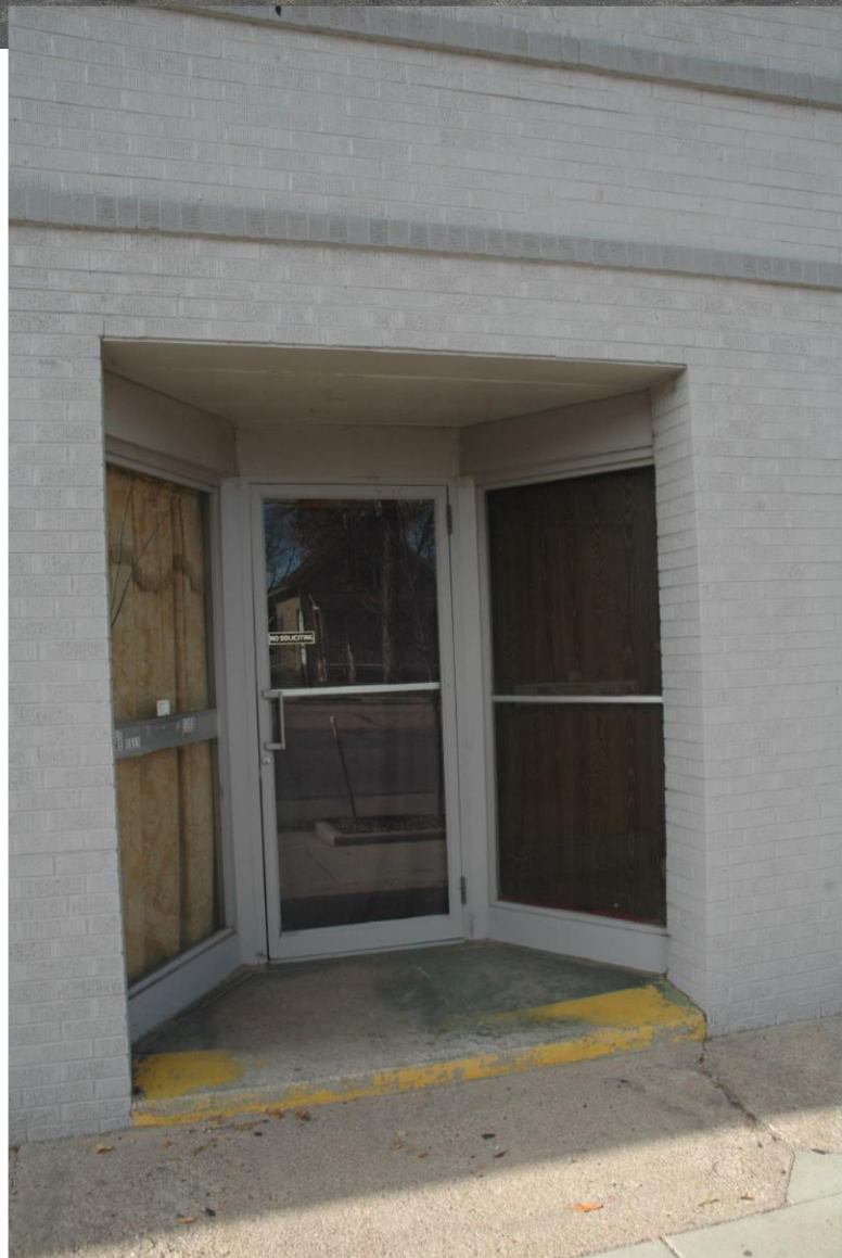
CD 1, Image 100, View to west of Recessed Entry on Facade
