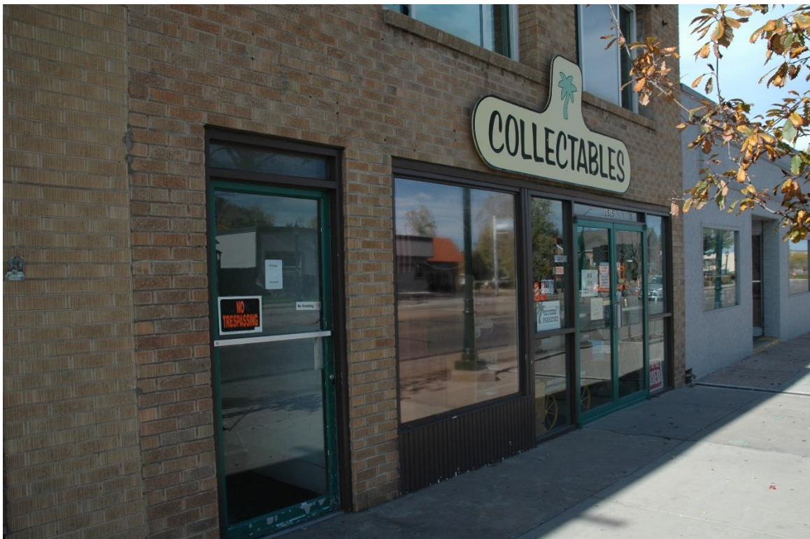
CD 1, Image 109, View to NW of lower facade
