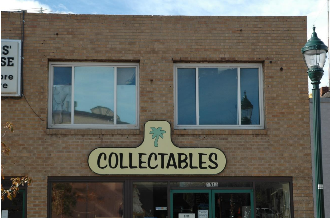
CD 1, Image 108, View to west of upper facade
