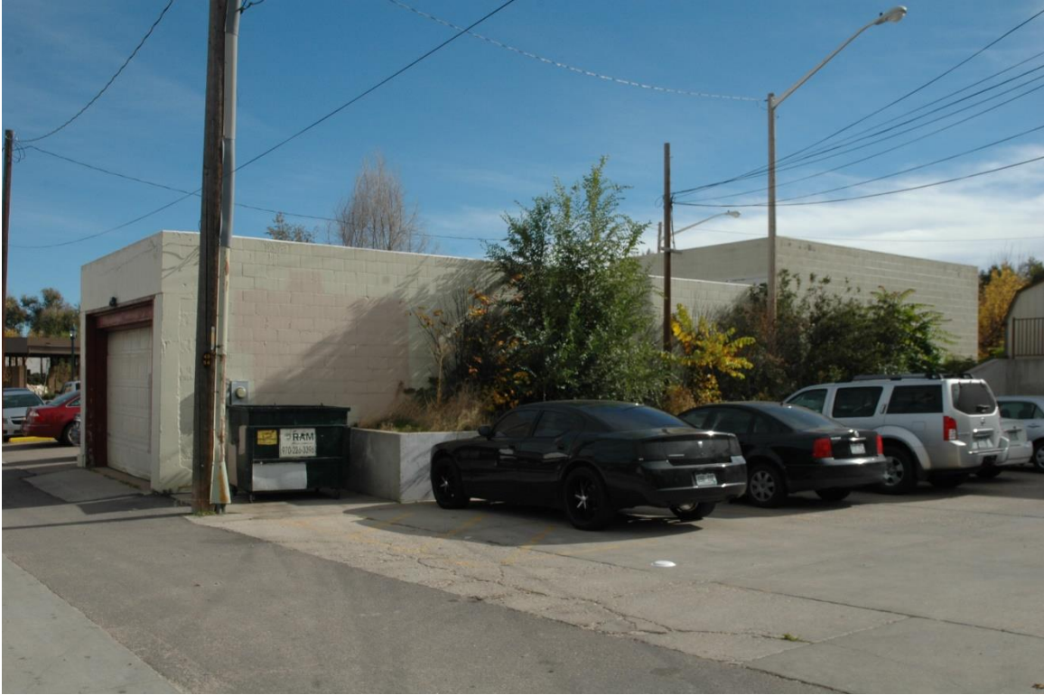
CD 1, Image 130, View to SE of rear additions (west)
