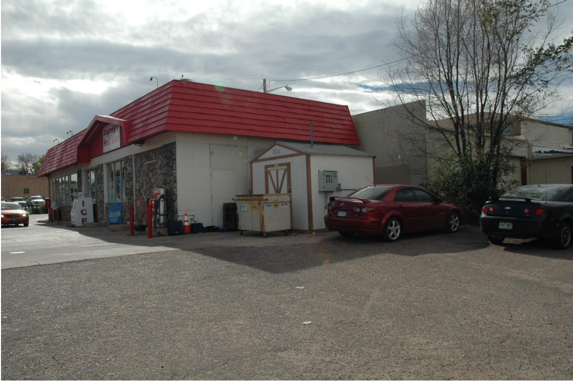
CD 1, Image 132, View to SW of façade (east) and north side
