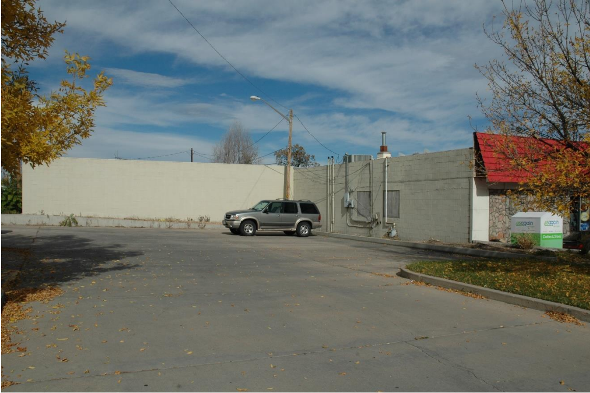
CD 1, Image 134, View to north of south side of rear additions
